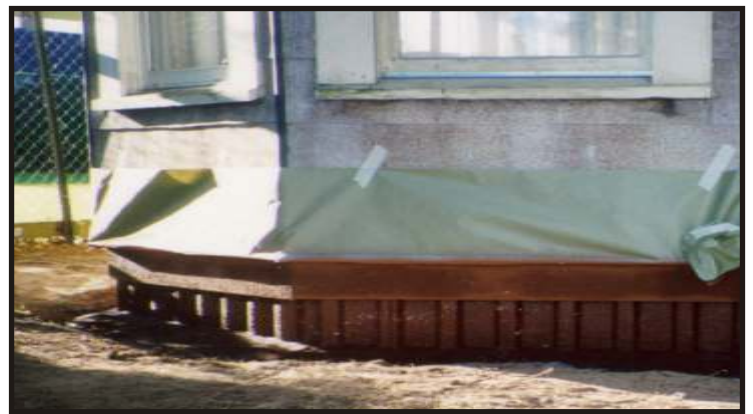
The ANCHORPANEL solution, as a cement-coat is drying.
