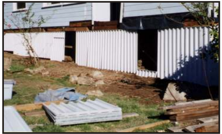
ANCHORPANEL low-cost retrofit foundation in progress.
