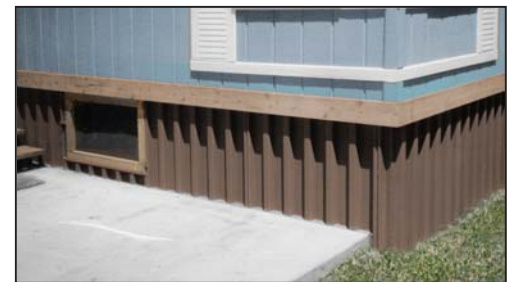
Pour concrete right up to it.
