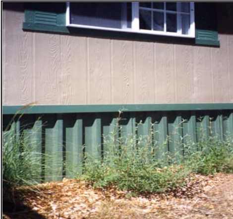
Apply cement color/texture coat.
