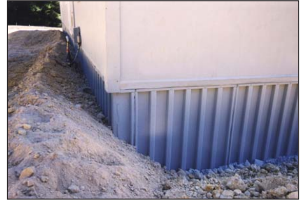
Cast in place panels can be back-filled against. Divert runoff water away from your home installation, keeping it nice and dry.
