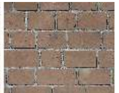
A stenciled-brick stucco finish.
