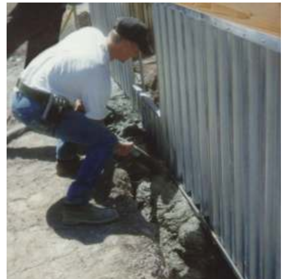
Placing concrete for a 2-story home.
